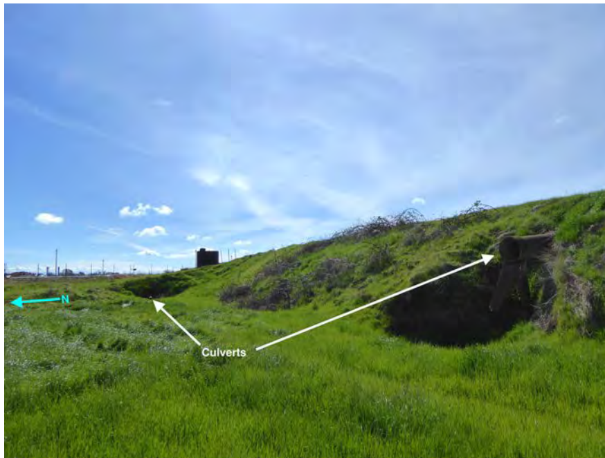
Water inputs to S parcel “detention basin”
